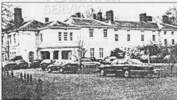
Conference centre Milton Hill House
